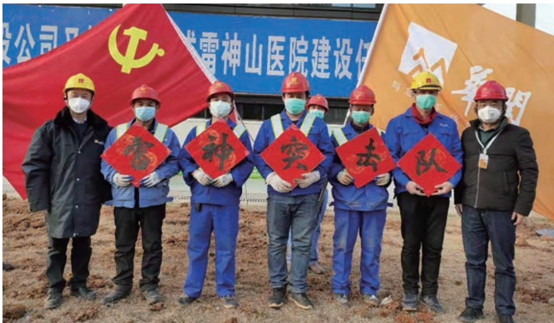
▲ 雷神山醫院成功通氣點火 Successful gas connection and ignition at Leishenshan Hospital
